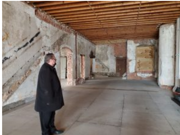
Developer David Ball shows off the empty interior of the recently renovated Pythian Castle. Photo credit: Sean Nestor.
